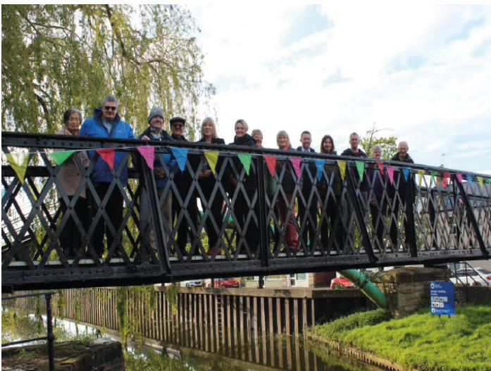
Saxilby Bridge refurbishment
